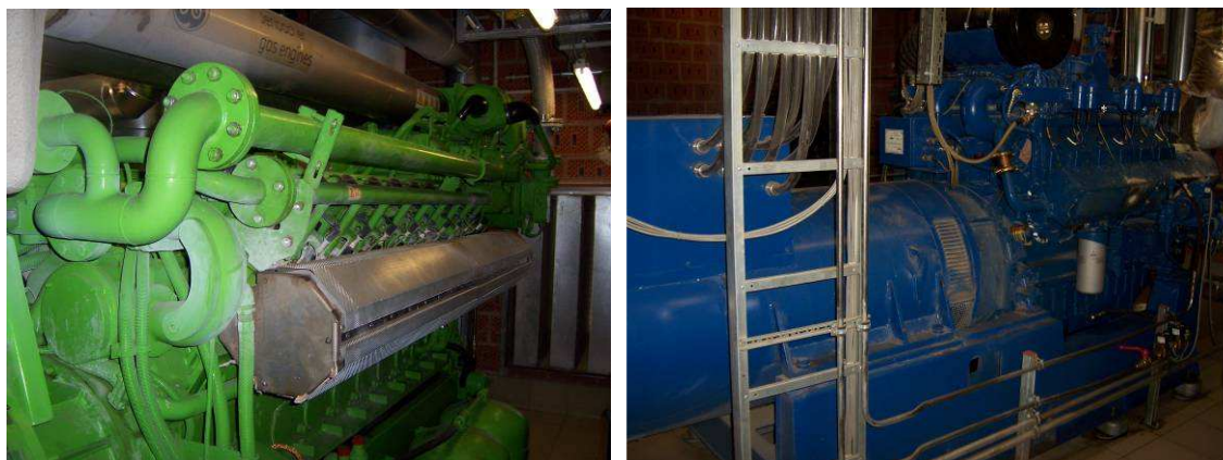
Figure 5.3 Gas-Otto engines (RUTZ 2007)
