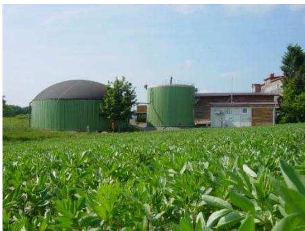
Figure 4.6 Vertical digester in Germany, processing pig and poultry manure and crop silage (KRIEG AND FISHER 2008)
