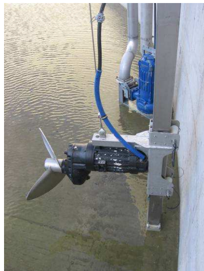
Figure 7.22 Submersible motor propeller stirrer (AGRINZ 2006)
