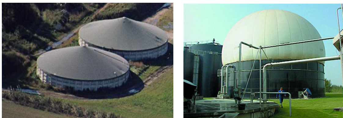
Figure 7.33 Membrane covered storage tanks (DANISH BIOGAS ASSOCIATION 2008)
