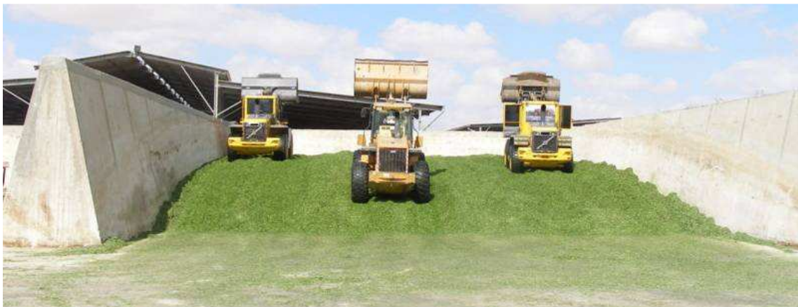
Figure 7.5 Bunker silo (WIKIPEDIA 2008)
