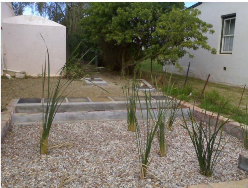
Figure 13: 4m 3 single household digester (in background), anaerobic baffled reactor (midground) and gravel filter (foreground) producing Water Affairs compliant water quality while processing sewage and food scraps to produce thermal energy for cooking (Source: AGAMA Biogas, 2007)
