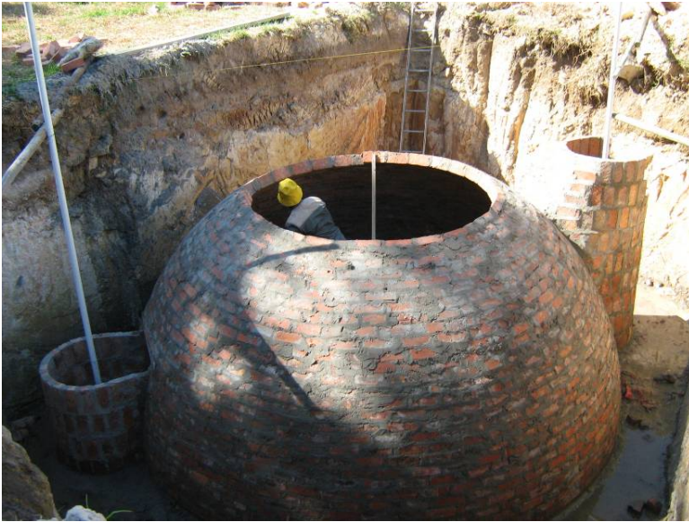
Figure 12: Construction of a 20m 3 biogas digester for processing sewage wastewater, food scraps and chicken litter (Source: AGAMA Biogas, 2007)
