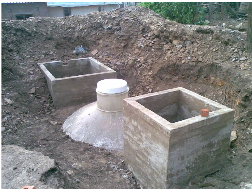
Figure 14: Construction shot of household digester for processing cattle manure, biogas produced fully offsetting fuel wood use and providing much needed fertiliser in the form of bioslurry to the garden (Source: AGAMA Energy, 2008).
